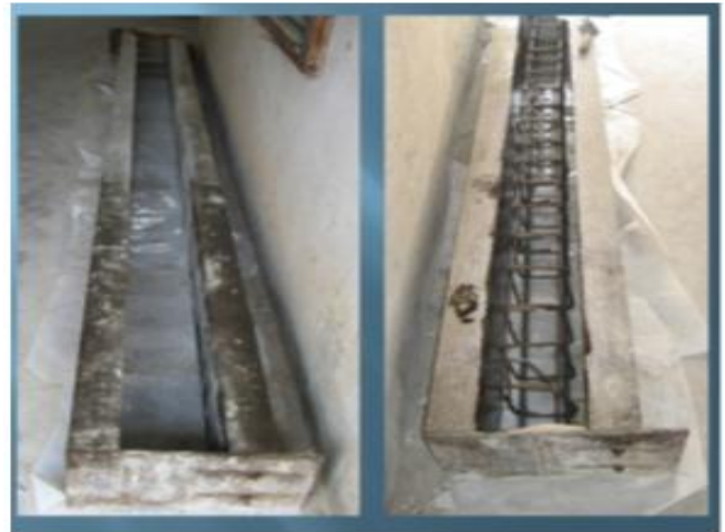
Fig3. Steel Frame Used For Casting of Beam.
